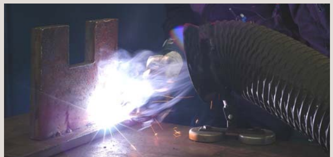
Use weld fume exhaust systems for improved working environment.
